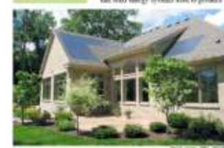
This home in Ohio uses a roof-integrated solar electric system to offset energy consumption.
