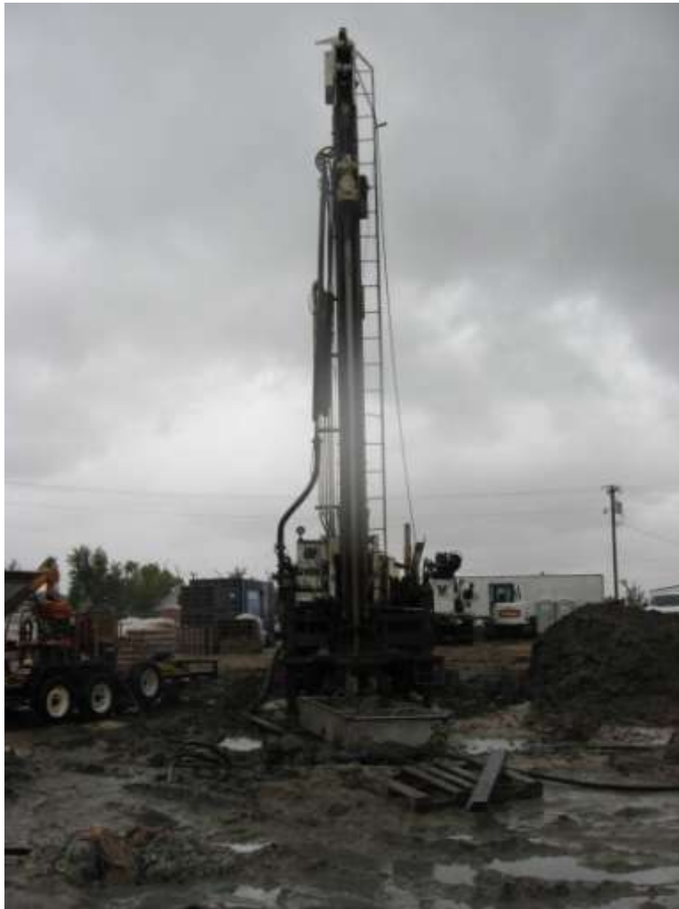
Drilling geothermal wells at the Courthouse
